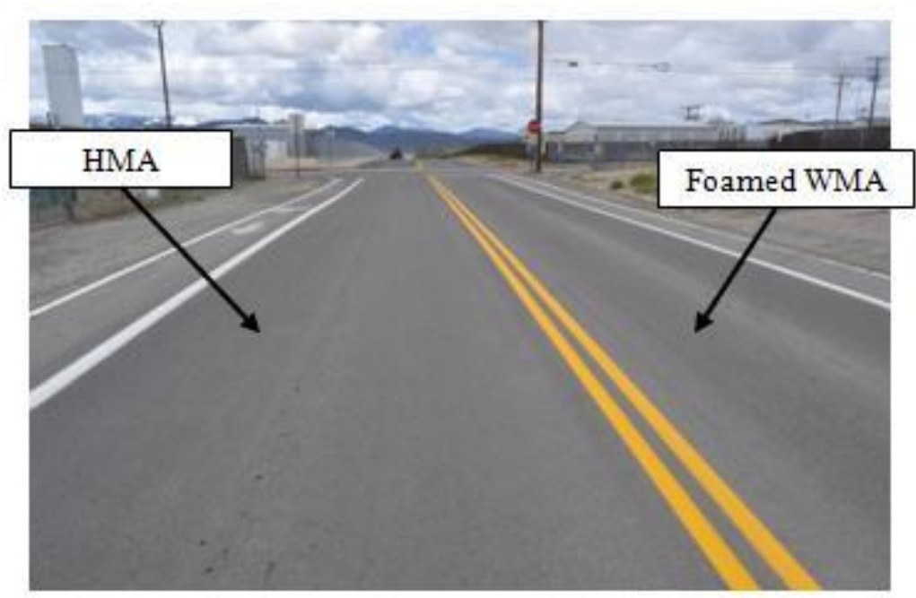
Figure 34 Photo for HMA and WMA Pavements on Bravo Avenue (May 18, 2011).
