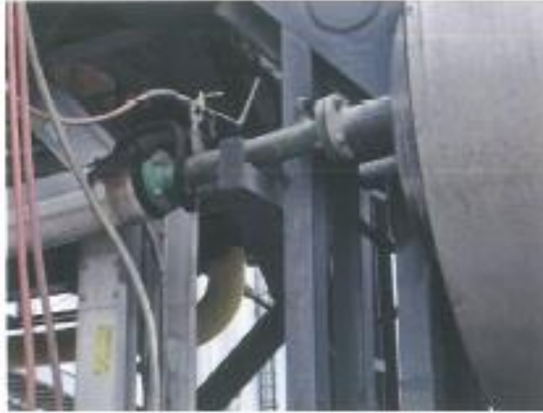
Figure 7 AquaFoam Foaming Unit Installed in Asphalt Line.
