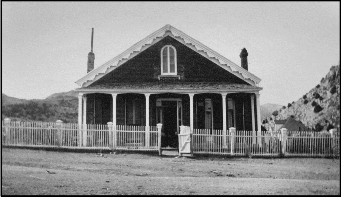
Figure 4.2. A picture of the Levy home taken ca. 1905. Note the decorative details such as the bargeboard, false balcony, gabled windows, and two chimneys. Image courtesy of the Nevada Historical Society.
