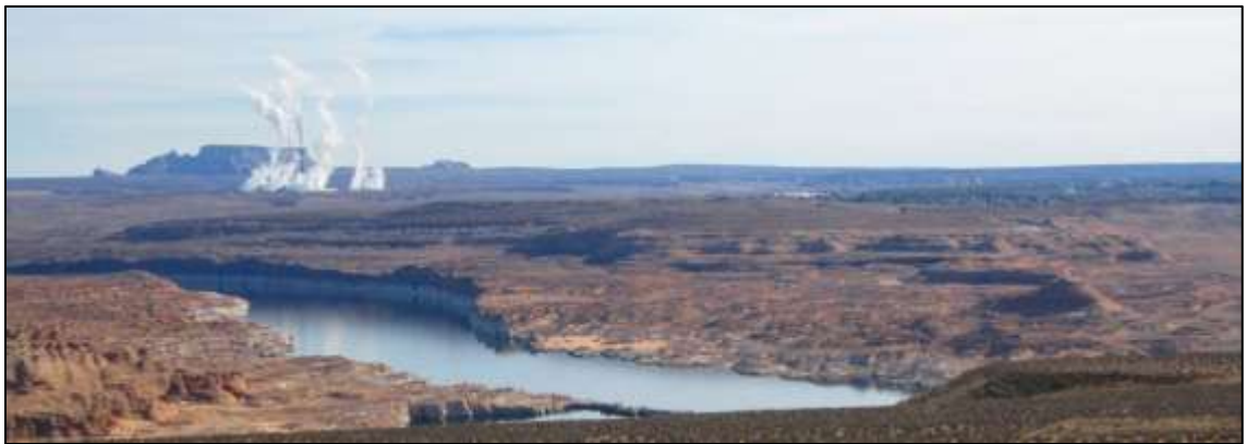
Figure 6: Navajo Generation Plant at Glen Canyon (2012). By K. Heslop.
