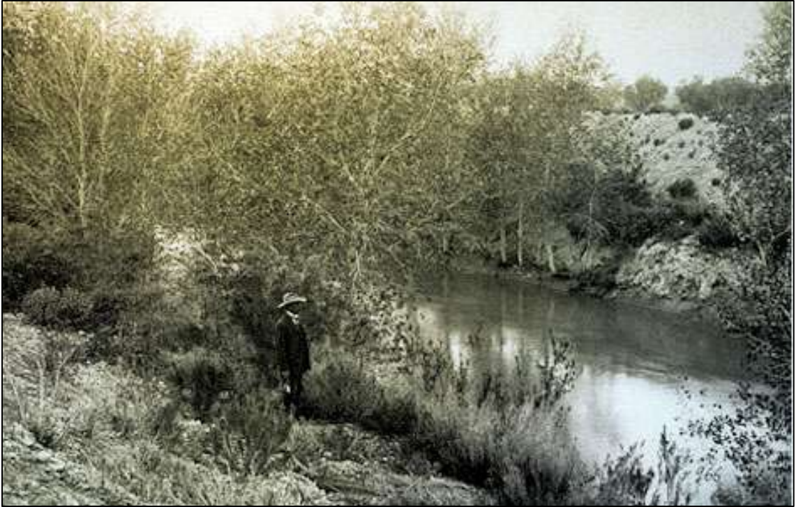
Figure 12: A prehistoric Hohokam canal has been incorporated into the Consolidated Canal in the eastern Salt River Valley (1906). Hand-tinted glass slide. Courtesy: Bureau of Reclamation
