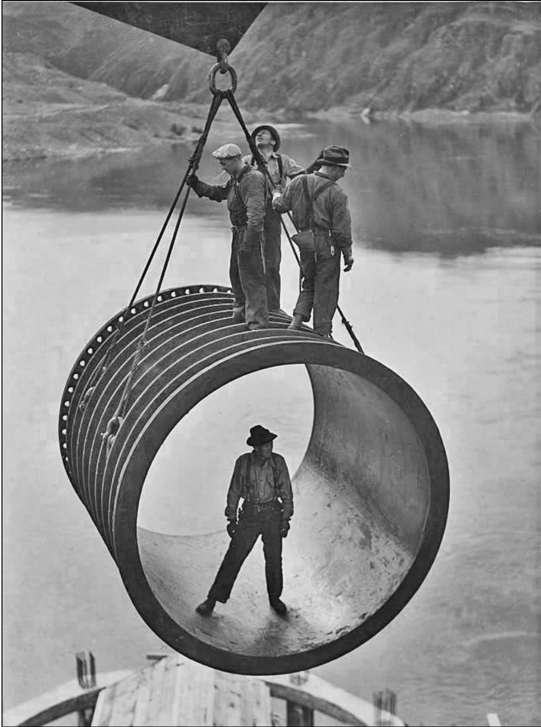
Plate 20: Four Men: three standing on top and one standing inside, riding on large casing section of pipe suspended by cable as it is moved into position by a crane, reservoir in the background during construction of the Grand Coulee Dam, Washington.
