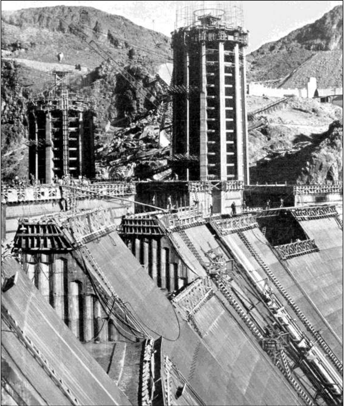
Plate 12: Construction Nears Completion, Boulder Dam.
