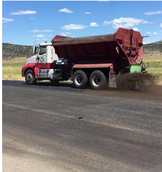
Figure 5.5. Photo. Distributor applying sand.
