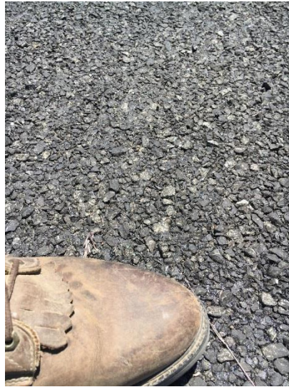
Figure 5.4. Photo. Final chip seal.
