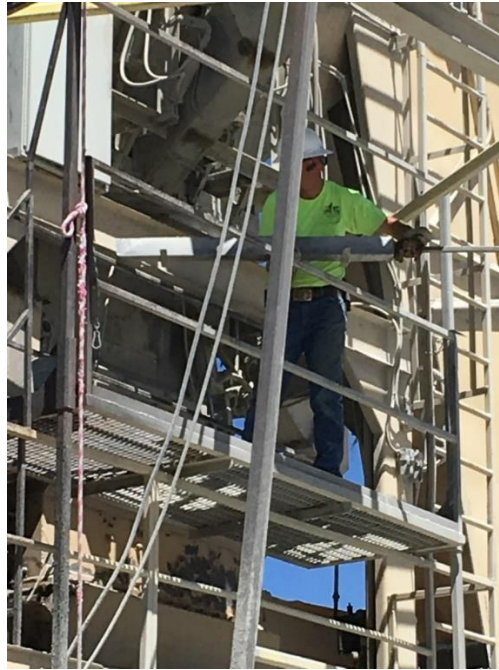
Figure 5.7. Photo. Pre-coated aggregate sampling
